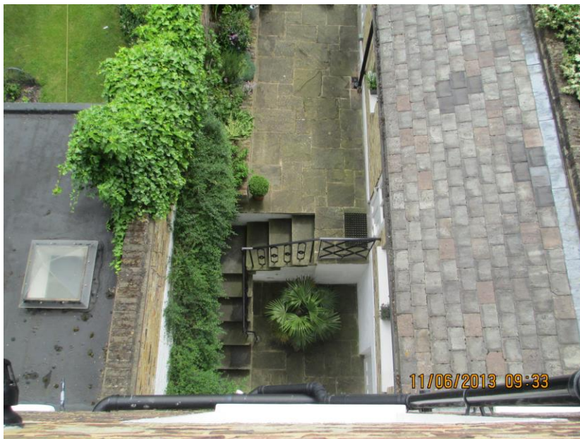
5. Looking down at the existing projection and basement area
