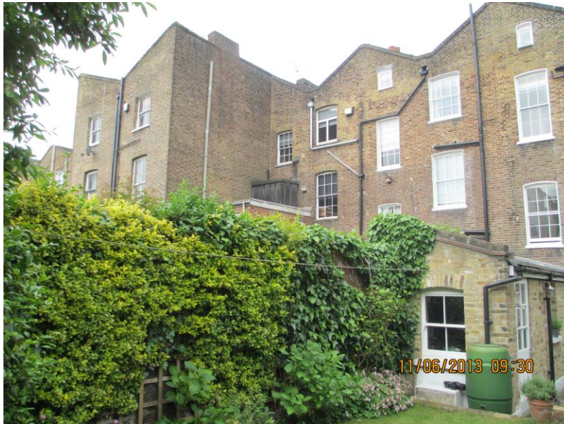
4. Looking towards number 104 Barnsbury Road
