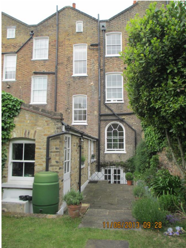
2. The rear of the property
